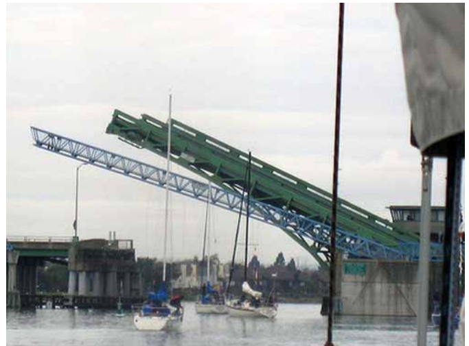
...which opens obediently for them to pass through. (The blue bridge is the separate bike path and was completed in 1995. How many working bicycle drawbridges are there in the USA, anyway? According to Alameda County, exactly ONE . Info at http://tinyurl.com/bikedrawbridge )
